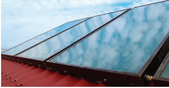
with an existing heating system without needing major modification of the building fabric – which is one of the reasons why solar thermal systems are one of the most widely used microgeneration systems in the UK.
