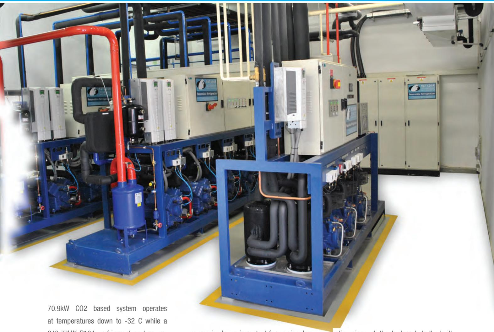
70.9kW CO<sub>2</sub> based system operates at temperatures down to -32 C while a 648.77kW R134a refrigerant system operates at temperatures at -10 C. Working together the two systems achieve cooling to a wide range of temperatures without using excessive energy or utilising CFC gases.
